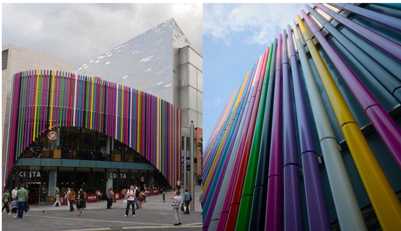
Colours applied are Ral 1023, Ral 3020, Ral 4003, Ral 4005, Ral 4006, Ral 4008, Ral 5002, Ral 5018, Ral 6018, Ral 9005 & Ral 9010
